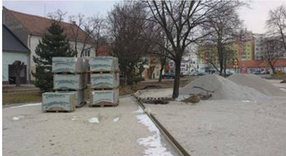
Figure 1 There is a high probability of the soil compaction and mechanical damage of roots due to storage of heavy material in the root zone of the tree
